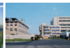
TBR Plant in Xiasha
